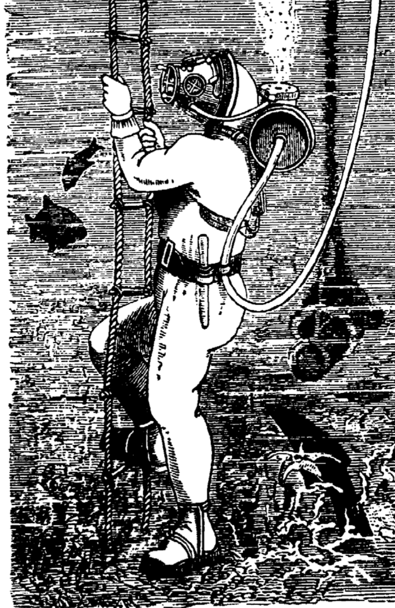
First published in the first (1876–1899), second (1904–1926) or third (1923–1937) edition of Nordisk Familjebok , this illustration shows a diving set developed by Rouquayrol and Denayrouze with a barrel-shaped bailout air tank on the diver's back
