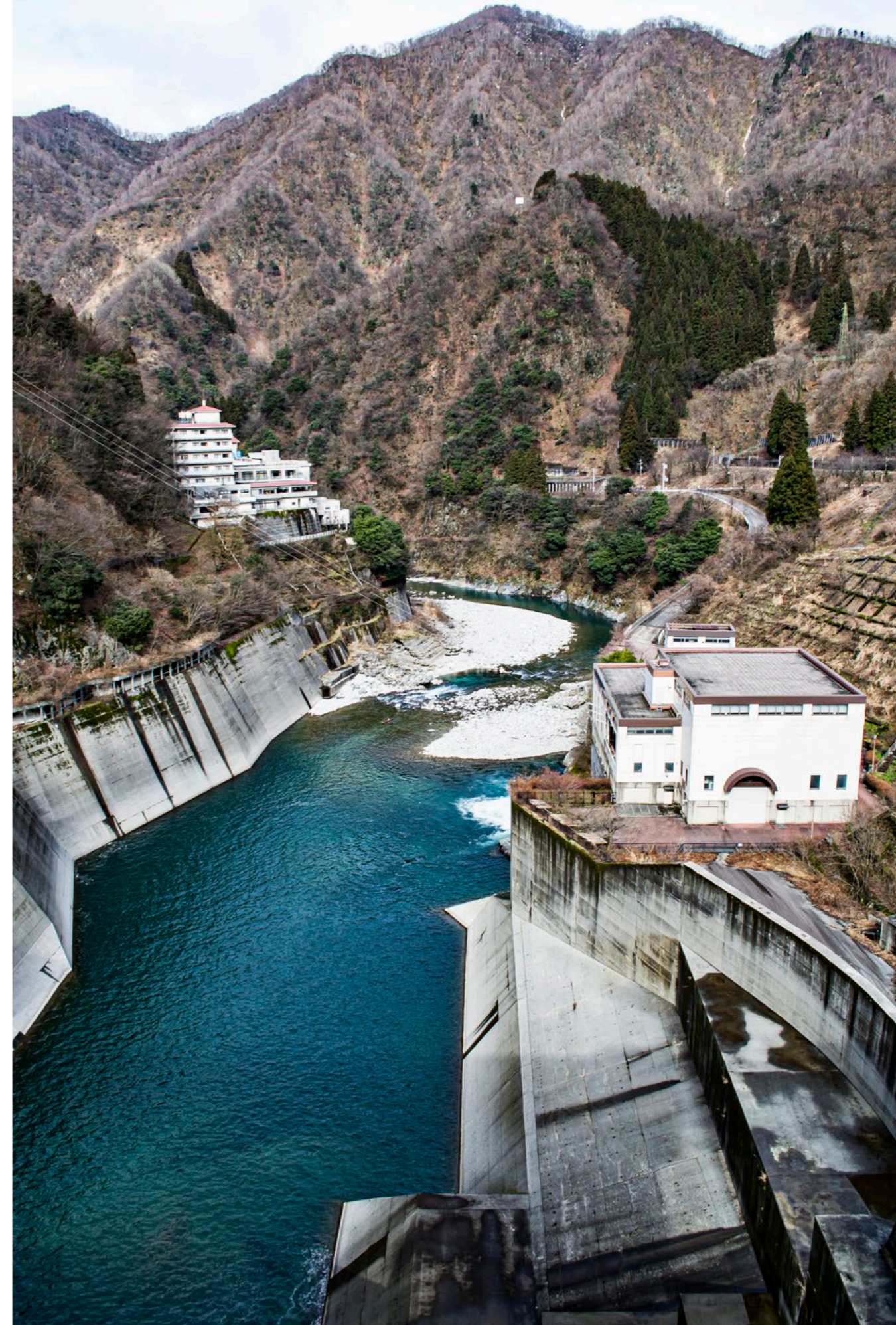
Dam of Toyama located in the mountains
