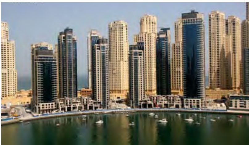
The Marina Promenade of Dubai under construction
