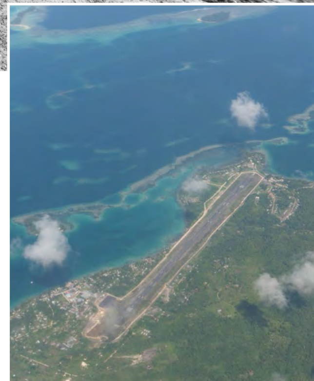
Munda Airport runway, constructed by the Japanese during WWII from October to December 1942; the United States captured the airfield in 1943.
